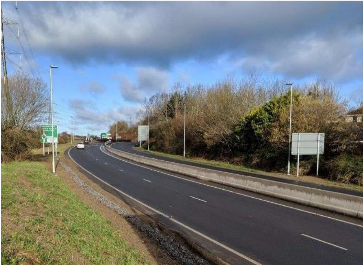
Previously dualled section of the Chippenham Bypass similar to current scheme
